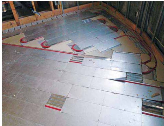
Lobodzinski improved the typical radiant heating with a rigid base and galvanized sheet metal in his Mammoth Lakes home.
