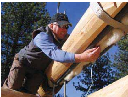
An installer uses lamb's wool to insulate the log grooves.
